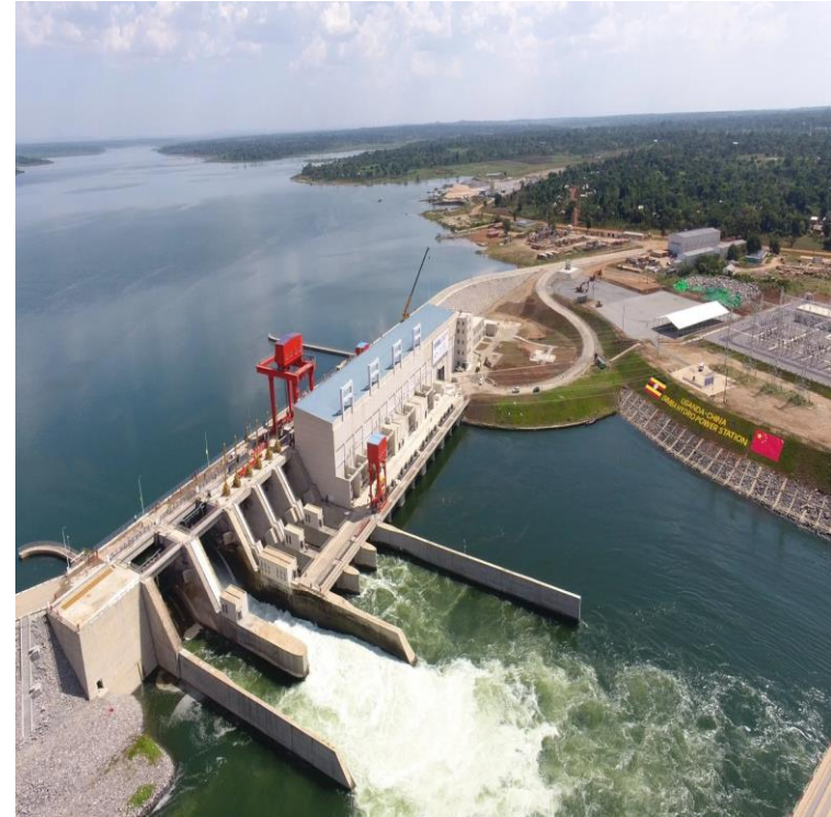
Isimba is a 183 megawatts Hydroelectric Power Station commissioned in 2019
